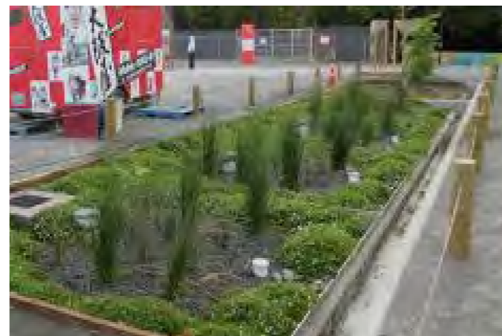
C - Carpark / road rain gardens
